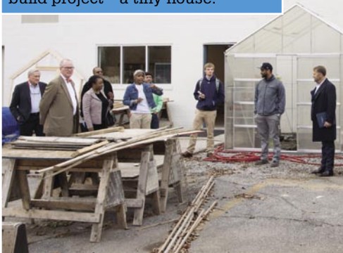
FROM THE INSIDE, OUT An Academy of Construction and Design tour starts in the classroom, (below) continues on the school's back lot and ends inside the latest build project—a tiny house.
